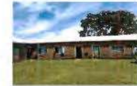
Structure to be demolished.
