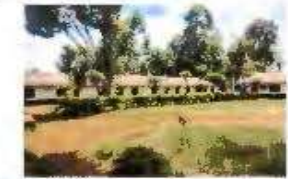
Existing structures to be demolished
