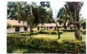
Proposed site - existing structures to be demolished
