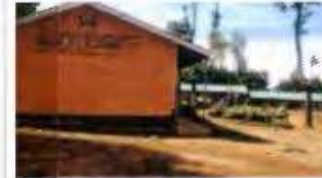
Classrooms refurbished by CDF
