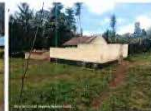
Sanitation facilities for staff.
