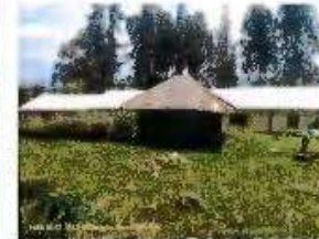
Existing Ntchen structure
