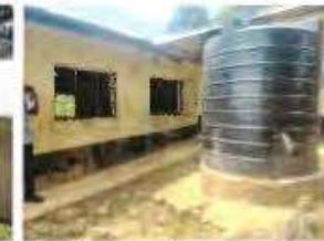
Rain water harvesting tank
