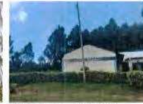
Existing administration and classroom block
