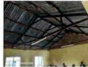
Roof structure in one of the classrooms
