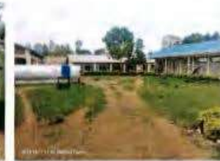
View of the existing administration block and classrooms
