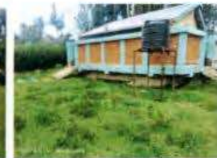
Elevated Pit latrine block; this prevents water from getting in when it floods
