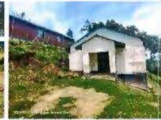
Abandoned dormitory block
