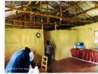
Administration offices with timber plywood partitions.
