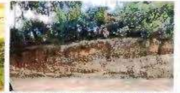
Difference between road level and site level
