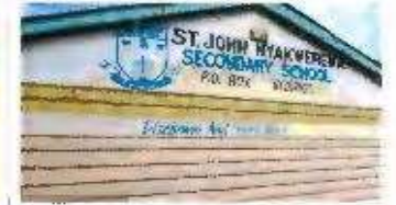
School administration block to be demolished
