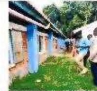
Existing classes to be demolished.
