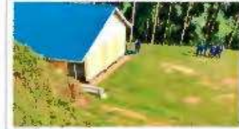
Existing classrooms below
