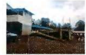
Proposed site of ongoing structure.
