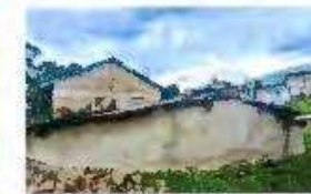
Existing water storage tank
