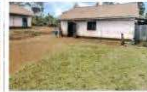
Existing ICT room
