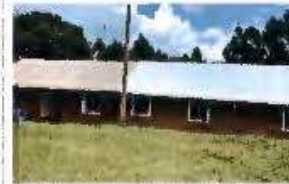
The variation of elevation on site demonstrating it's sloppiness
