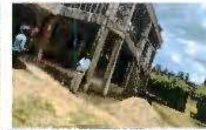
Different view of existing construction
