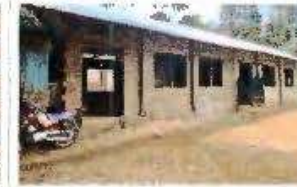
State of classrooms
