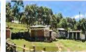
Pit latrines present in the school
