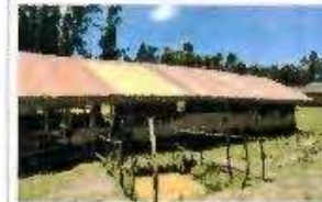
State of classrooms
