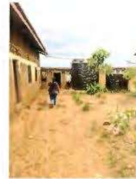
walk way and water storage tanks
