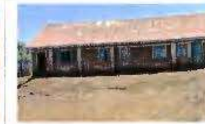
State of the existing class rooms
