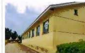
Side view of existing classrooms
