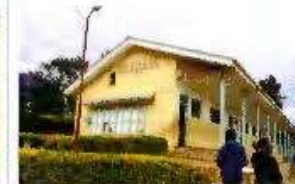
Front view of existing classrooms
