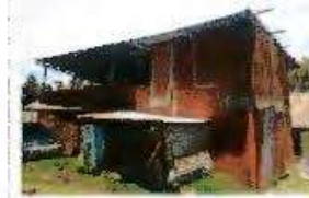
School bus shed to be demolished
