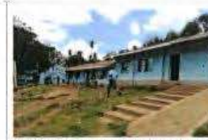
Existing classes to be demolished
