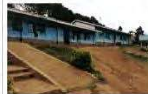
Existing classes to be demolished.
