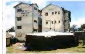
Dormitory and water storage tank
