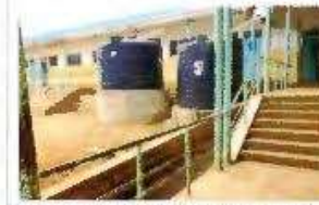
Walkway and water storage tanks
