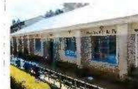
Existing dining to be demolished
