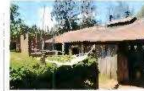
Existing kitchen that requires expansion
